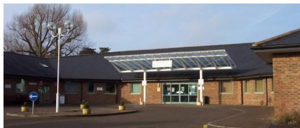
18 - Chepstow Community Hospital opened in 2000 having been developed under the Government's Private Finance Initiative.
